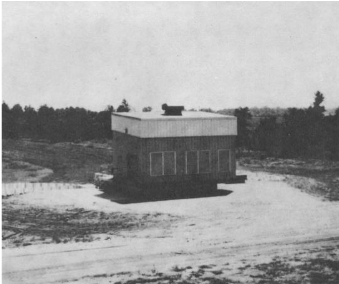
Photograph 10. Drinkwater Pumping Station -- Typical Agriculture Pumping Station
