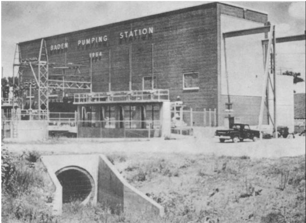
Photograph 8. Baden Pumping Station -- Early Major Pumping Station
