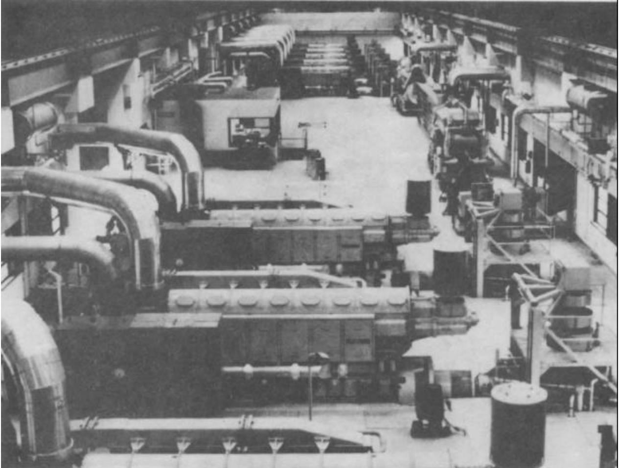
Photograph 2. W.G. Huxtable Pumping Station -- Interior View
