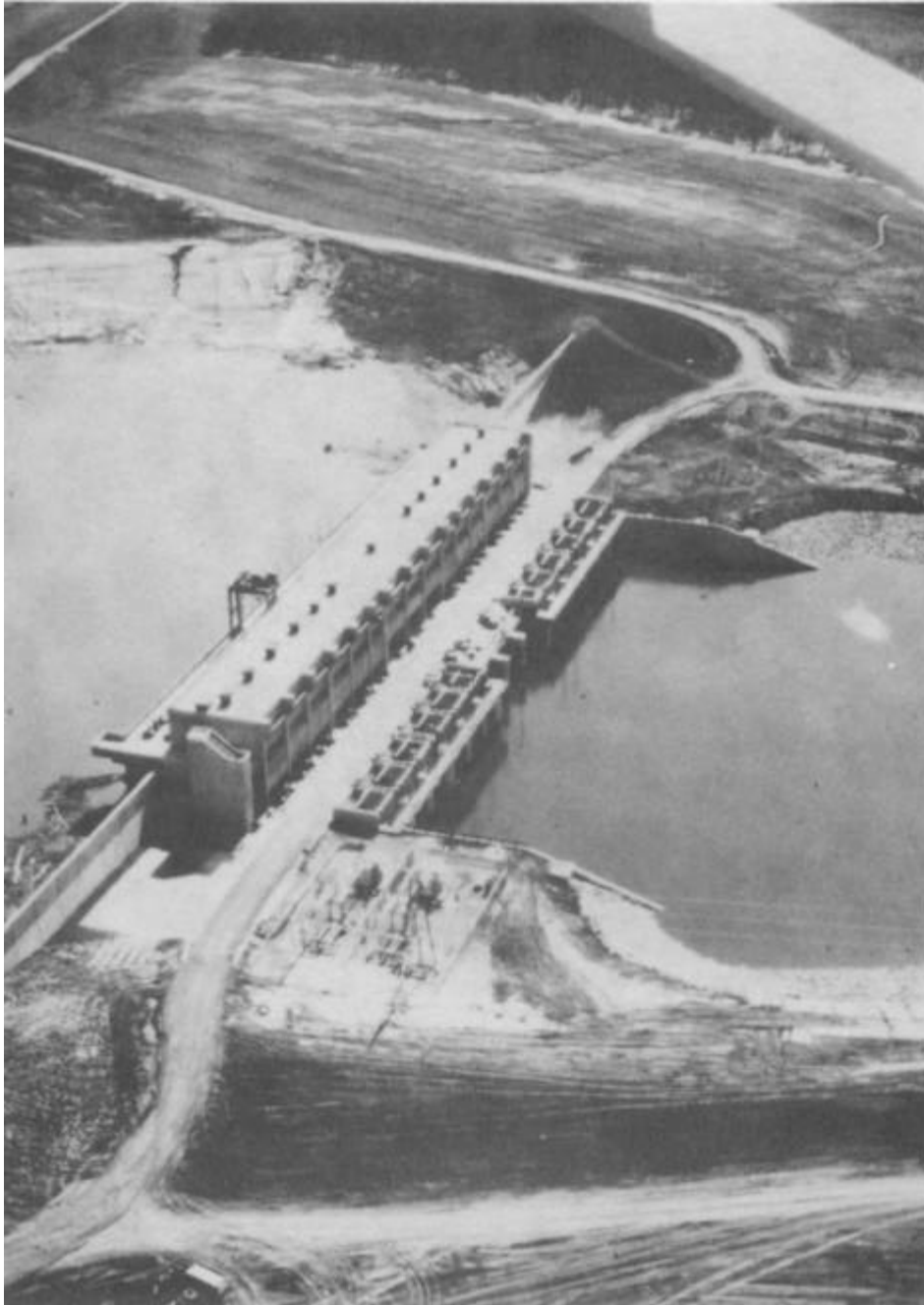
Photograph 3. Lake Chicot Pumping Station -- Aerial View
