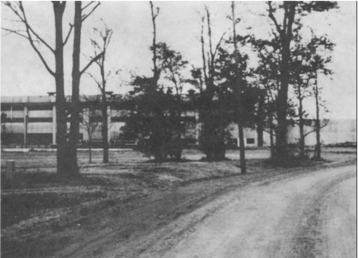
Photograph 6. Lake Chicot Pumping Station -- Blending Structures with Environment
